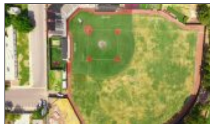
A project on a 40 by 40 foot site on New Mexico State's baseball field aimed to find out if artificial turf uses less water than real grass. (Ahmed Kanaan photo)
